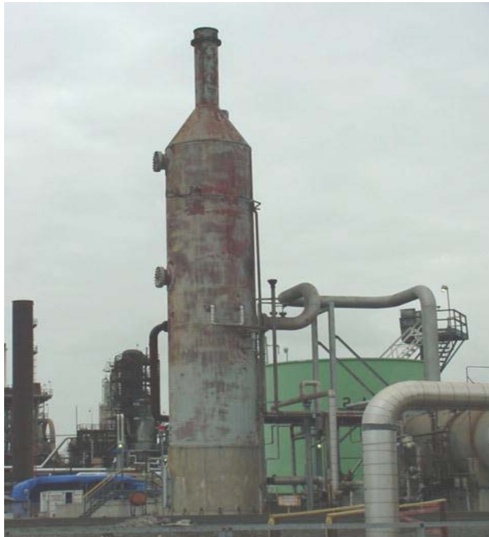
Figure 2: Crude Unit 3 Blowdown System
