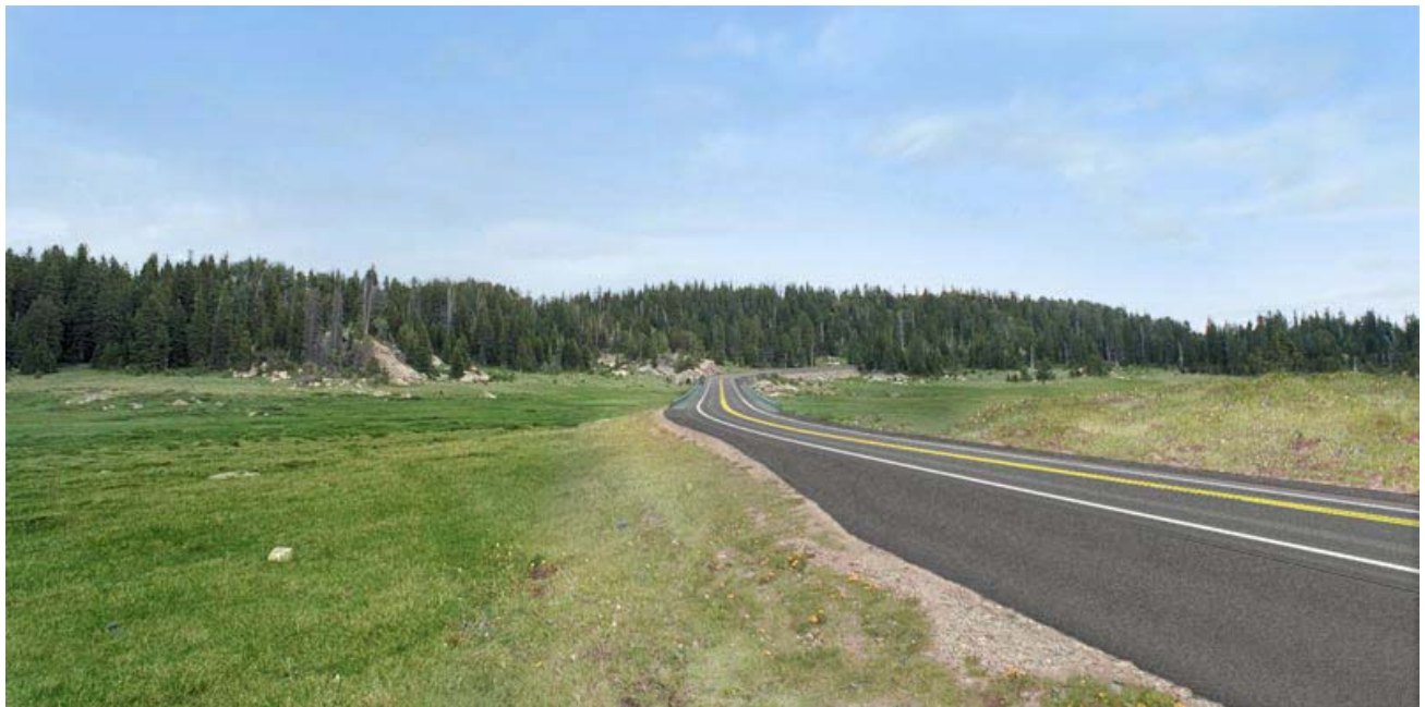
Visual simulation of a 9.6-m (32-ft.) roadway with pullout in foreground; the preferred alternative would have a 9.0-m (30-ft.) roadway at this location. Not shown in the simulation is a proposed bridge across Little Bear Lake fen.
