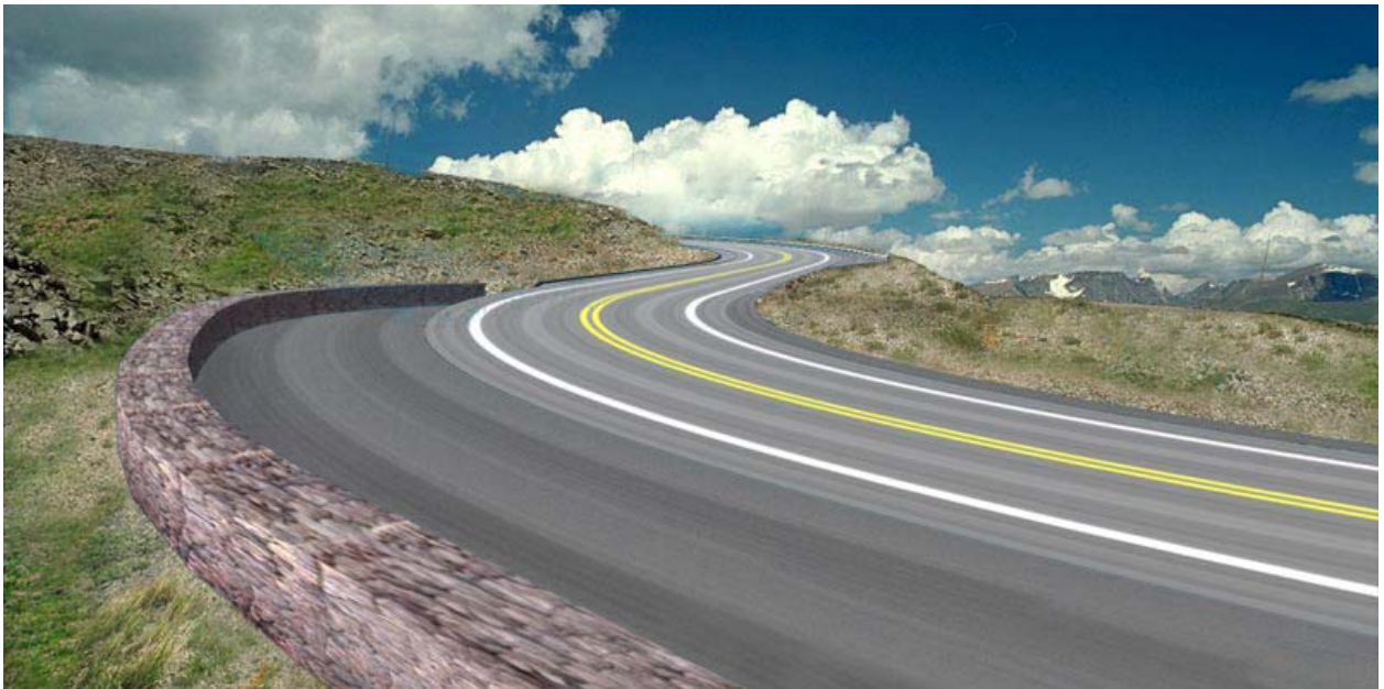
Visual simulation of a 9.6-m (32-ft.) roadway with a proposed Bar Drift parking area in the foreground. The preferred alternative would have an 8.4-m (28-ft.) roadway width at this location.
