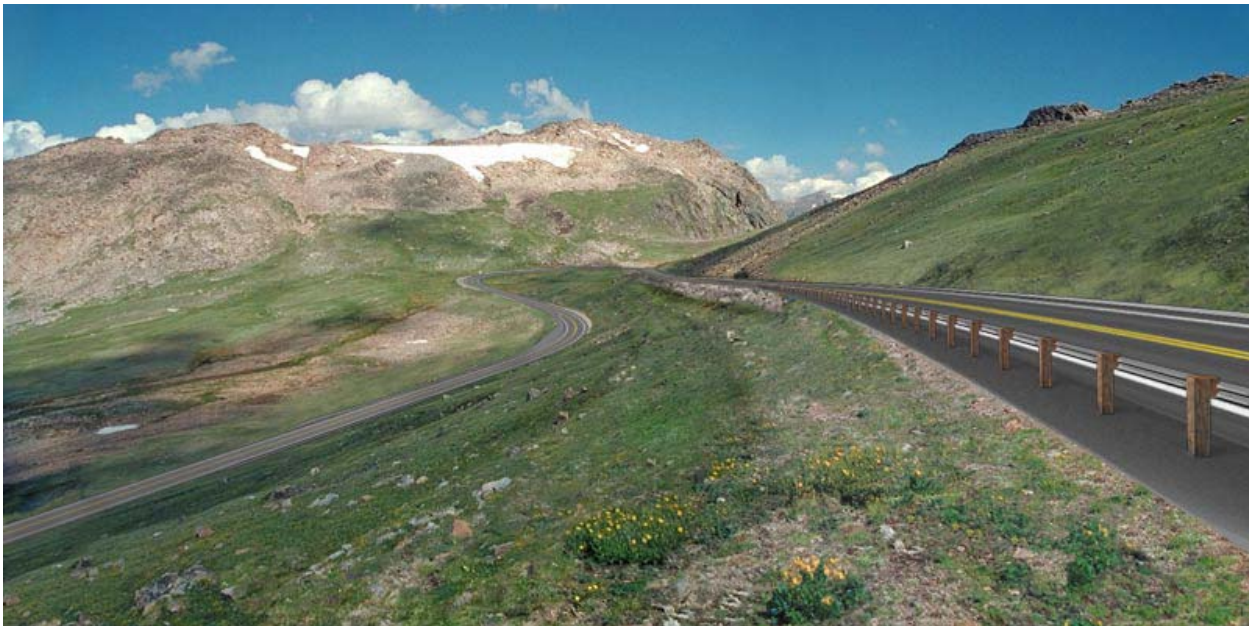
Visual simulation of a 9.6-m (32-ft.) roadway; the preferred alternative would have an 8.4-m (28-ft.) roadway width at this location. Guardrail would be needed where the adjacent slopes are steep.
