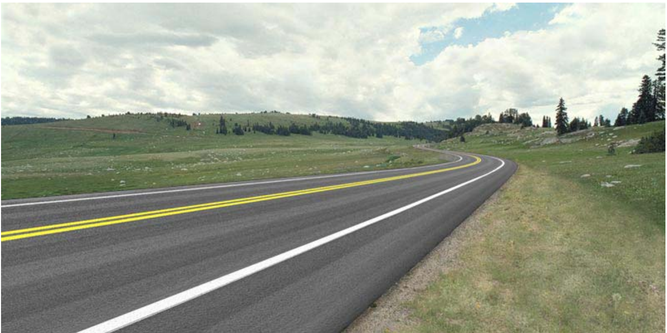
Visual simulation of a 9.6-m (32-ft.) roadway; the preferred alternative would have a 9.0-m (30-ft.) roadway at this location.
