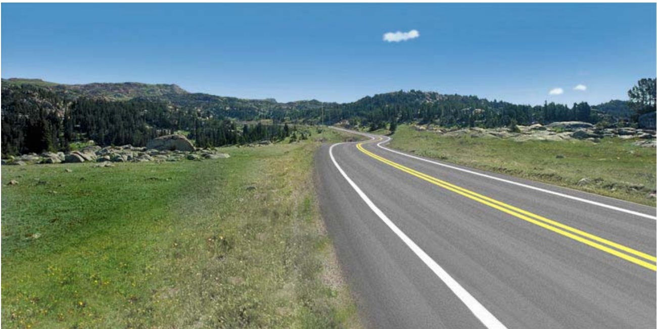
Visual simulation of a 9.6-m (32-ft.) roadway; the preferred alternative would have a 9.0-m (30-ft.) roadway width at this location.
