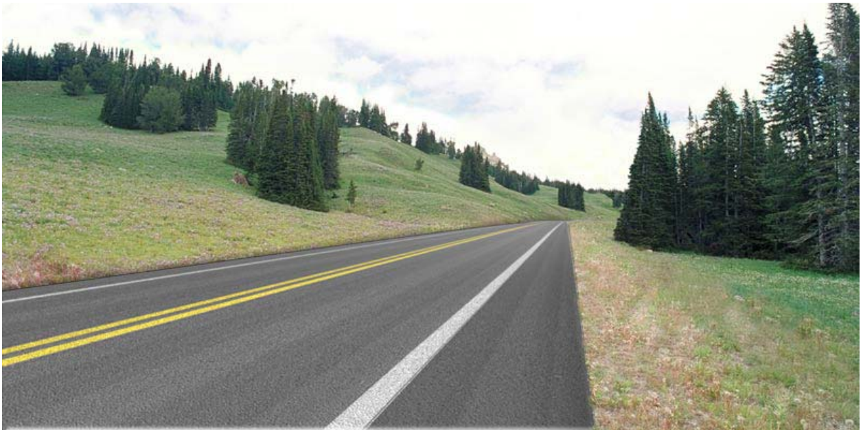
Visual simulation of a 9.6-m (32-ft.) roadway; the preferred alternative would have a 9.6-m (32-ft.) roadway at this location as a transition to a 9.0-m (30-ft.) roadway at Clay Butte Lookout turnoff.
