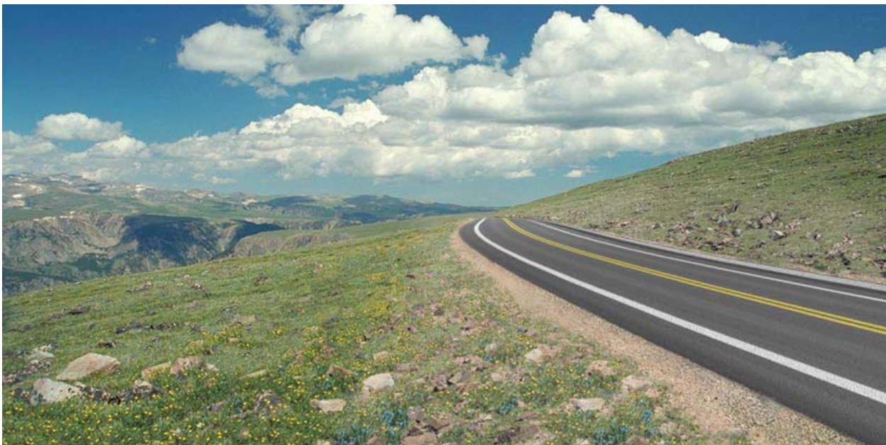
Visual simulation of a 9.6-m (32-ft.) roadway; the preferred alternative would have an 8.4-m (28-ft.) roadway width at this location.
