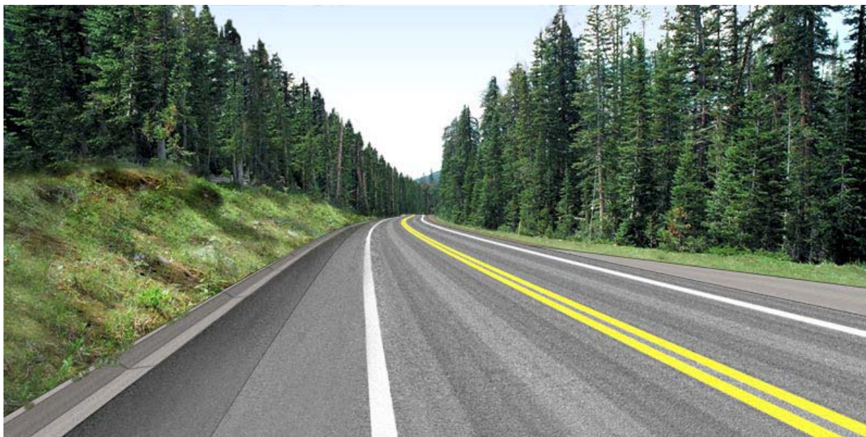
Visual simulation of a 9.6-m (32-ft.) roadway; the preferred alternative would have a 9.0-m (30-ft.) roadway at this location. A paved ditch with curb would eliminate ditch erosion and minimize cutslope disturbance.
