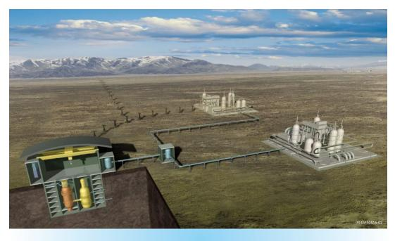
The Very-High Temperature Reactor could produce both electricity and heat for hydrogen production.
