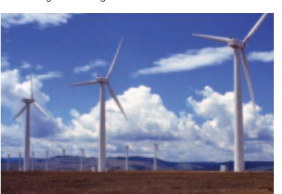
**Hull Municipal Lighting Plant** — The **Hull Municipal Lighting** Plant (HMLP) installed its first wind turbine—a Vestas 660-kW V-47 machine—in December 2001. Located at the end of the peninsula in Hull, Massachusetts, the turbine is estimated to produce 1.5 million kilowatt-hours of electricity each year. One-third of the output provides electricity for Hull's streetlights and traffic signals. The
