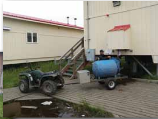
Typical village “haul” system. Water delivery trailer and sanitation holding tank. Photo credit: Jennifer Dobson
