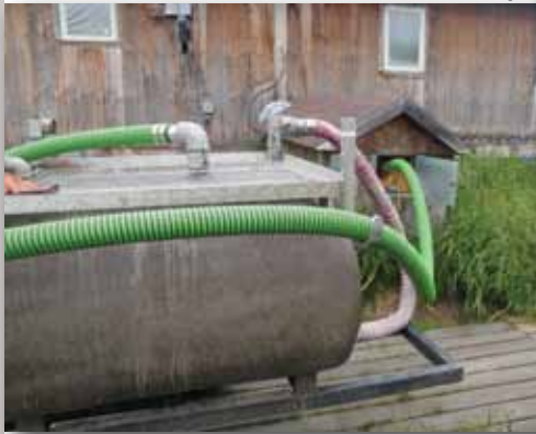
Typical village “haul” system. Water delivery trailer and sanitation holding tank. Photo credit: Jennifer Dobson
