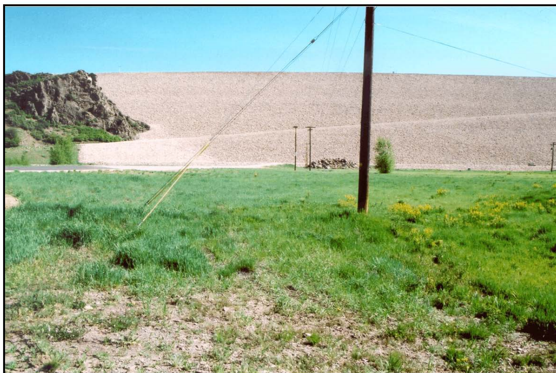
Figure 3. Overview of the project area; view to the north.
