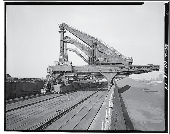
A Hulett Ore Unloader before its removal as part of the Pennsylvania Railway Ore Dock project in Cleveland (photo courtesy Library of Congress)
