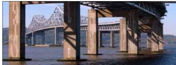
This view of the existing Tappan Zee Bridge shows the innovative floating caissons in the foreground. (photo courtesy Wikipedia Commons)
