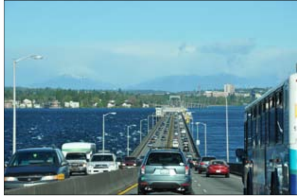
Evergreen Point Bridge over Lake Washington, located on Interstate 5 in Seattle, is slated for replacement. (Photo courtesy Washington Department of Transportation)
