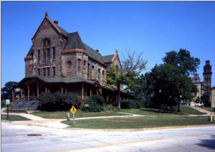
Ward Memorial Hall, or Building 41, at the Clement J. Zablocki Veterans Affairs Medical Center (Photo courtesy HABS/HAER collection, Library of Congress)
