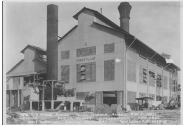
The larger portion of the structure is the power plant which will remain a contributing element, and the smaller structure to the left houses the boiler, which will be removed. (Photo courtesy U.S. Navy)
