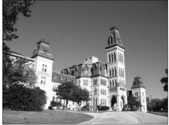
Old Main, or Building 2, at the Clement J. Zablocki Veterans Affairs Medical Center (Photo courtesy HABS/HAER collection, Library of Congress)
