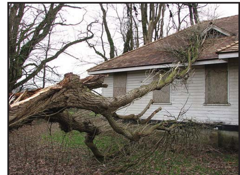
Tree damage from storm event
