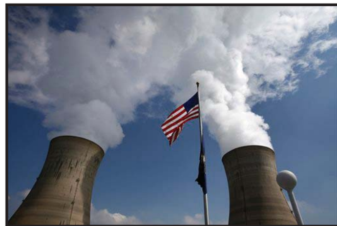
Nuclear cooling towers
