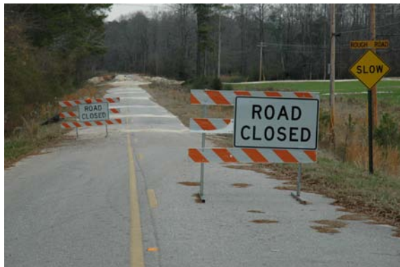
Road closed due to sinkholes
