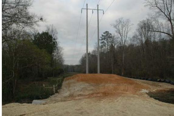
Power lines moved because of sinkholes / soil instability
