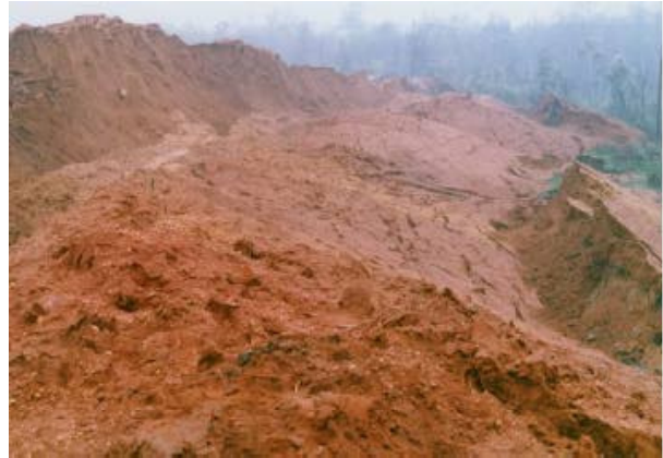
Figure 5.22 A Land Slide in Alabama
