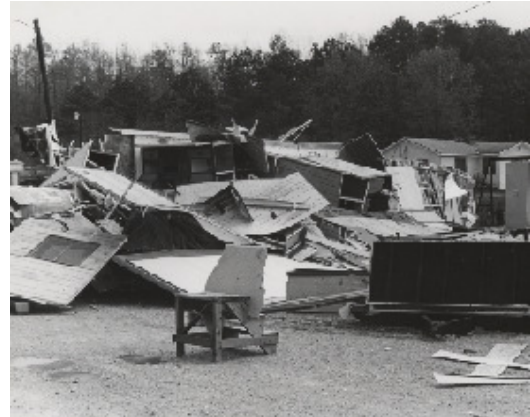
Figure 5.19 Pelham Alabama 1973 Tornado Shopping Center Damage
