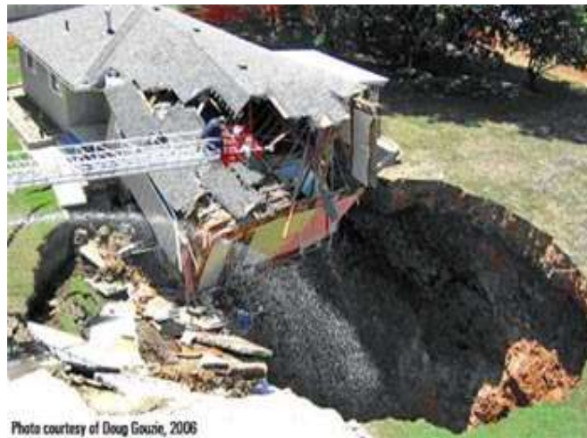
Figure D-11. Sinkhole Collapse of House
