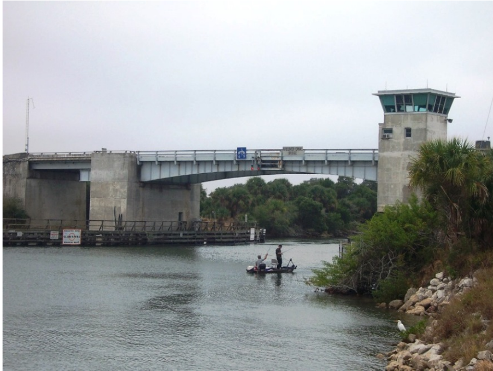
Figure 2.1-8. Haulover Canal Bridge
