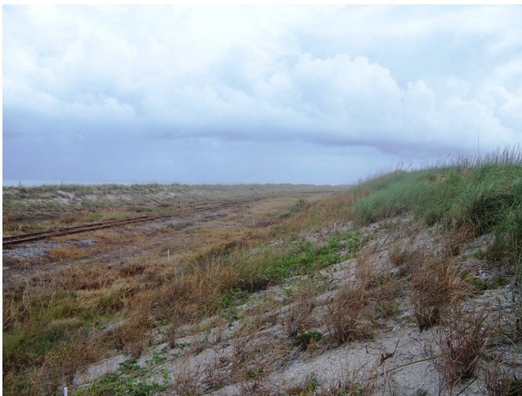
Figure 3.7-5. Coastal sand dunes at KSC provide a protective barrier between damaging waves, seawater and infrastructure
