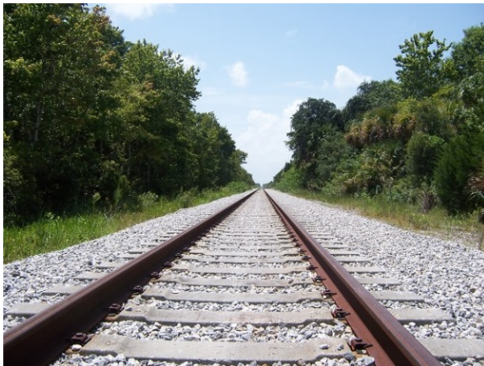
Figure 3.12-1. Railroad tracks at KSC and MINWR
