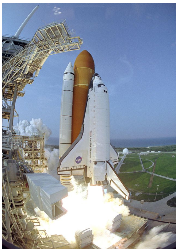
Figure 3.10-1. LC-39 – Pad A is one of several facilities at KSC listed on the NRHP
