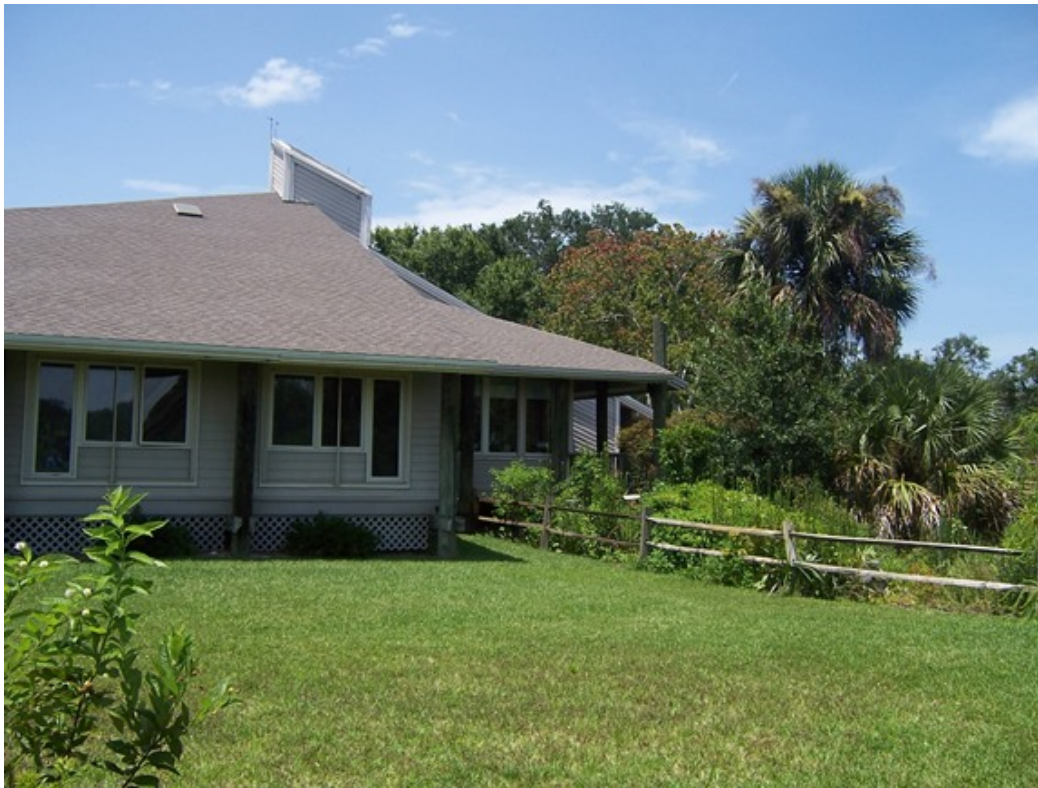
Figure 3.15-2. Visitor center at MINWR
