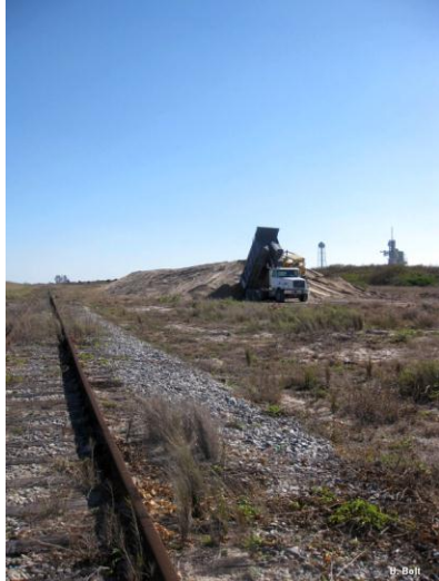
Inland dune construction, Aug. 2010
