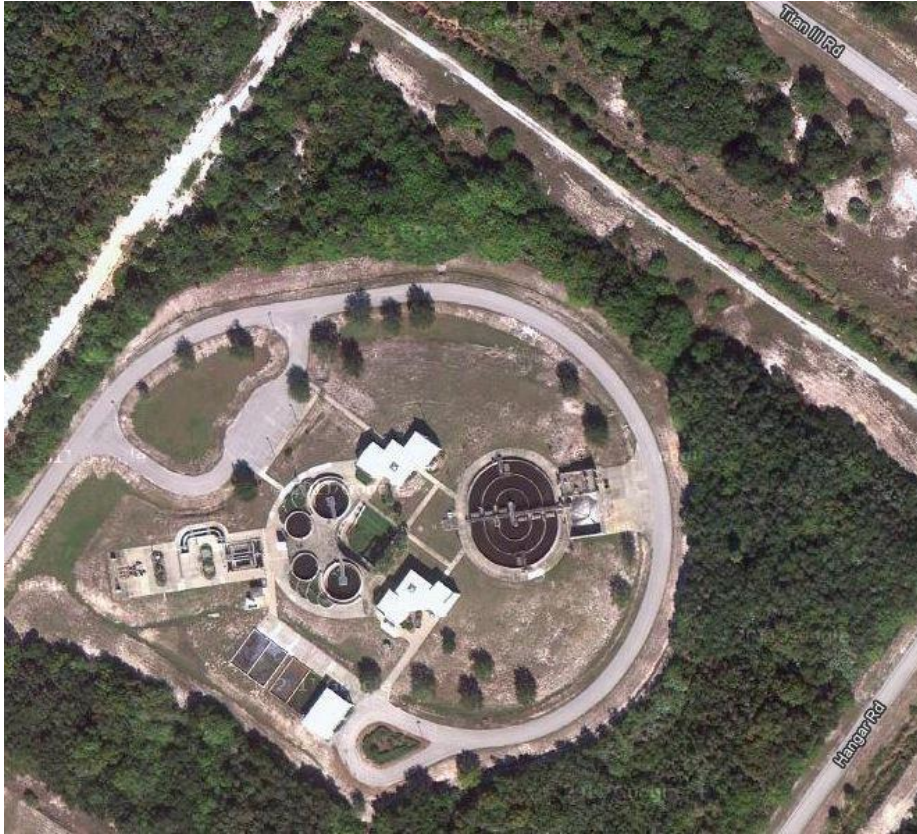
Figure 73. CCAFS waste water treatment facility.
