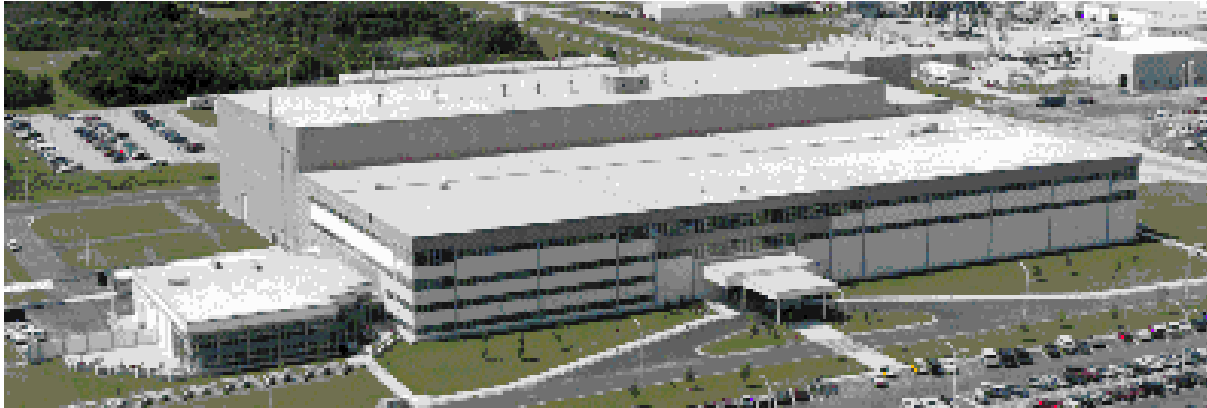
Figure 72. Aerial view of the SSPF built to support testing and verification and integration of Space Station hardware and modules. Construction of this facility initiated programs to restore and create habitat for the federal protected Florida Scrub-jay.
