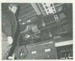
...Jim Garvey adjusting frequen of the nuclear magnetic resonan probe, in service building A2...
