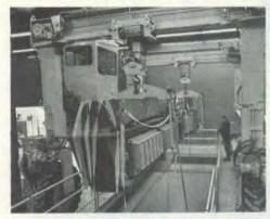
....Cross Gallery "travel-lift" machine lowers 48th girder, supporting final two Booster magnets....
