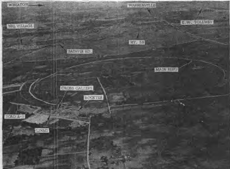
An Autumn, 1969 aerial view of the National Accelerator Laboratory site, looking east-south-east. Excavation and clearing work outline the Main Accelerator and the road inside it. The Linac, Booster and Cross Gallery are at the lower left. The NAL Village is above and to the left of the Main Ring. Wheaton, Warrenville and The East-West Tollway are at the top of the view. (Photo by Don Mendenhall, NAL)
