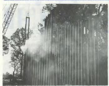
.... Sheet-piling work on the beginning of the Proton Laboratory....
