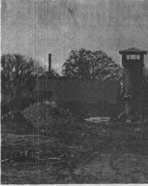
A silo on the former Schimmelpfennig farm has become the NAL "observation tower" during the construction phase of accelerator system. The tower stands on the southern perimeter of the Booster ring. The DUSAF construction office is located nearby.
