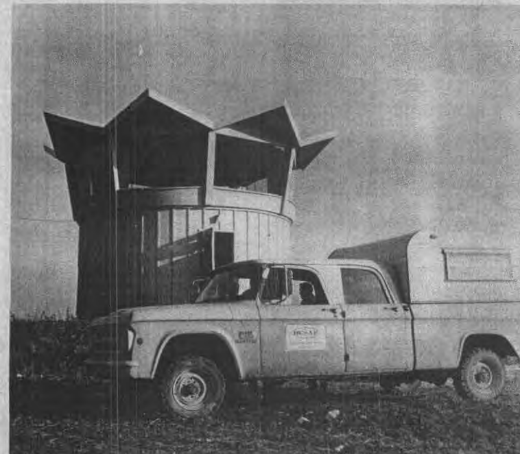
"The Gazebo," the NAL Survey Tower, was developed by DUSAF and stands in the precise center of the Main Ring. It is elevated about 25 feet and the upper section rotates
