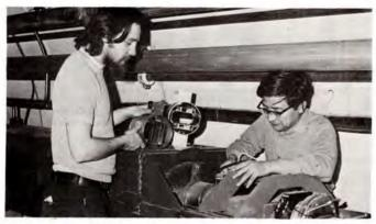
...Bob Pighetti (L) and Ryuji Yamada installing position detector plates inside the vacuum chamber in the main ring tunnel...
