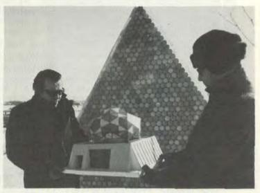
....Main Ring's Bob Sheldon (left) shows model of translucent, honeycomb effect of proposed Bubble Chamber geodesic dome to Hank Hinterberger, NAL Technical Services. Dome will be made of discarded beverage cans....
