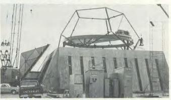
4) Steel frame was erected on top of Bldg. A as a base for the 3.8 ton completed sections which were raised by cables attached to cranes..
