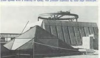
3) Next stages of assembly took place adjacent to Building A, shown in background. Circular crane now used in assembly work extended over top of building.
