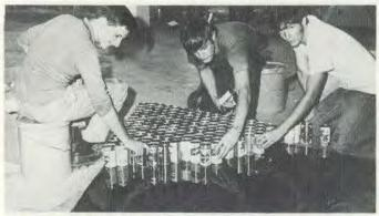
Each panel, a triangular "sandwich" of 2 slices of polyester-reinforced fiberglass spread with a coating of epoxy, was pressed together by sand bags overnight.
