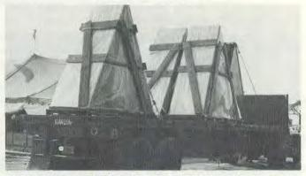
2) Crew of 5 men assembled 120 panels at rate of 6 per day. Fanels were moved from the assembly area to the bubble chamber area by truck..
