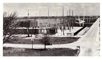
...Fermilab Master Substation. Foreground, left, capacitor tree to level peak demands from accelerator at 500 BeV...
