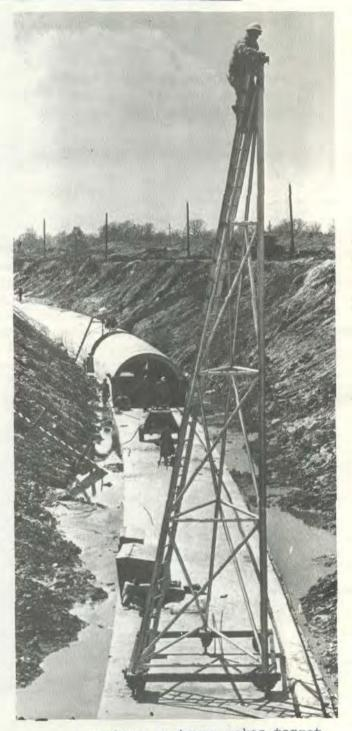
A workman on tower makes target adjustment for laser beam, used as a modern surveying device in construction of NAL's Main Accelerator enclosure. (Chicago Sun Times photo)
