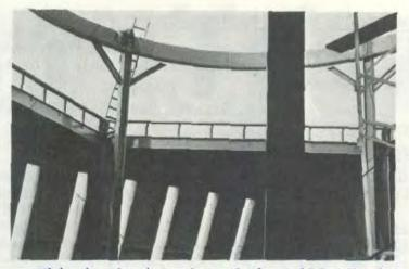
...This is the interior of the Bubble Chamber assembly building near completion near McChesney and Wilson roads on the NAL site. The man at the top is working on the circular-crane rails. The dome of this building will be constructed of panels of used beverage cans between fiberglass sheets...
