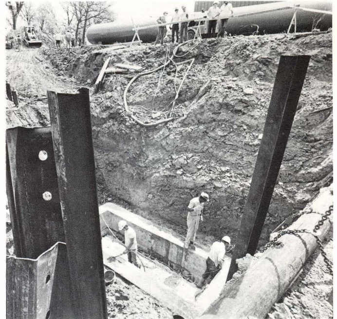
...In Switchyard upgrading, workmen install access shaft to beam line tunnel...
