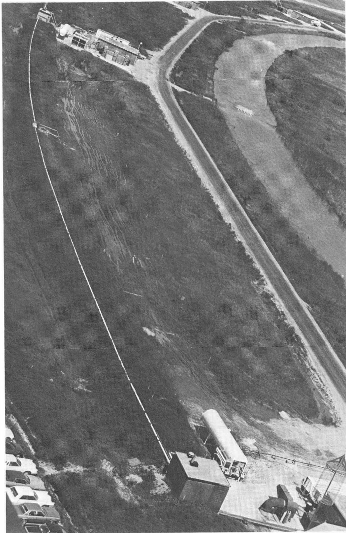
Helium transfer line running from A-1 service building (bottom of photo) to A-2 service building.
