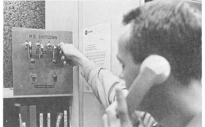
Mark Flaherty, Communications operator, demonstrates how he is able to shut off power to a stuck elevator upon receiving an emergency call.
