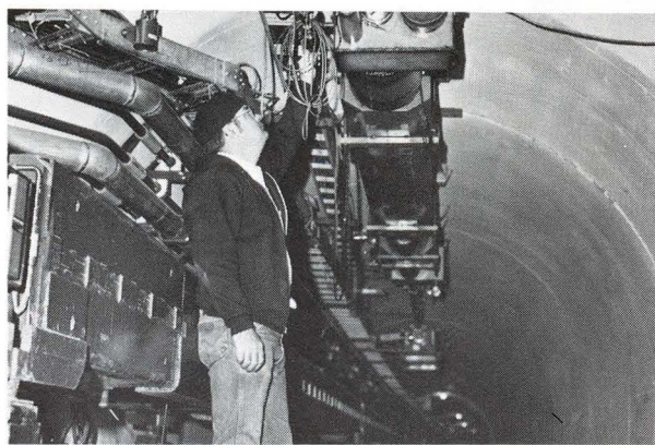
...Ron Norton at doubler prototype in Main Ring tunnel...
