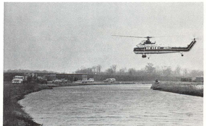
...Helicopter crosses main ring cooling ditch to pick up another load...
