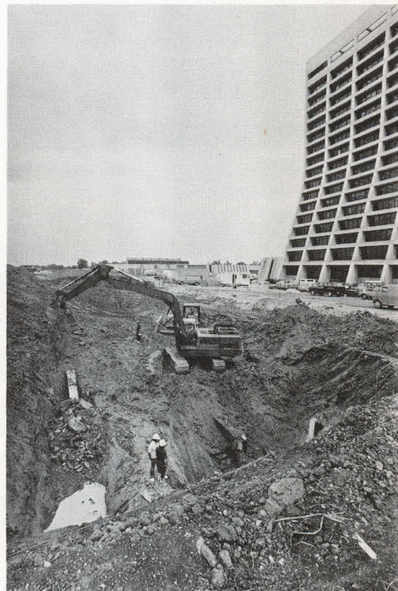
...Central Laboratory (east) overlooks transfer hall work...
