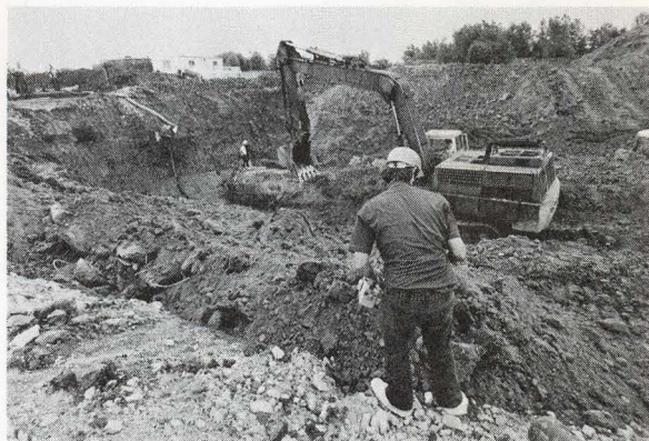
...Power shovel strips berm from beam pipe...
