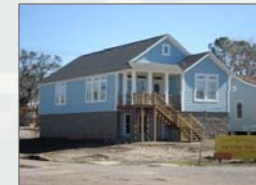
Extended Foundation Walls
