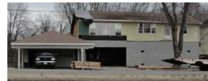
Branson, Mo. Substantially damaged April 2011 w/ 1 foot of flood water. Elevated to 1 foot above BFE (±8 feet).
