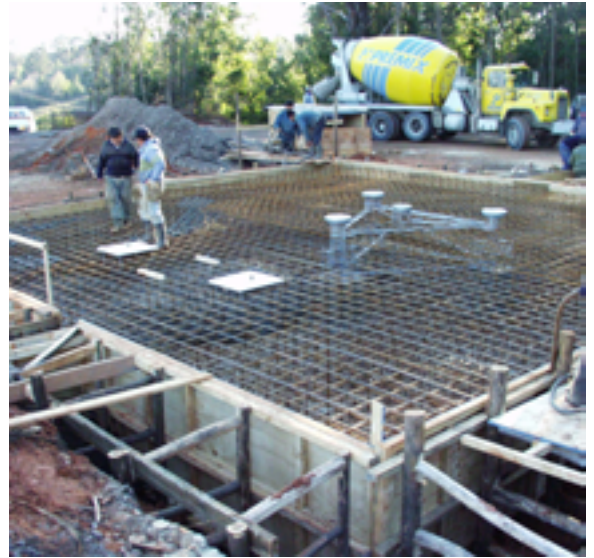
Future TIGO platform prepared for pouring the concrete.
