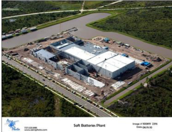
Figure II- 3: Saft Factory of the Future under Construction
