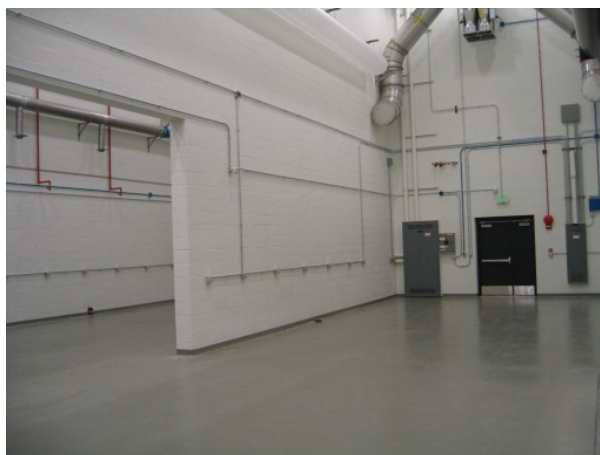
Figure IV - 248: MERF High bay, soon home to the Cathode Materials Scale-up Lab.
