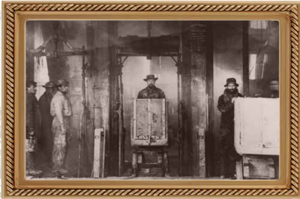
(Above) Curtis Shaft, Savage Mine, Virginia City.
