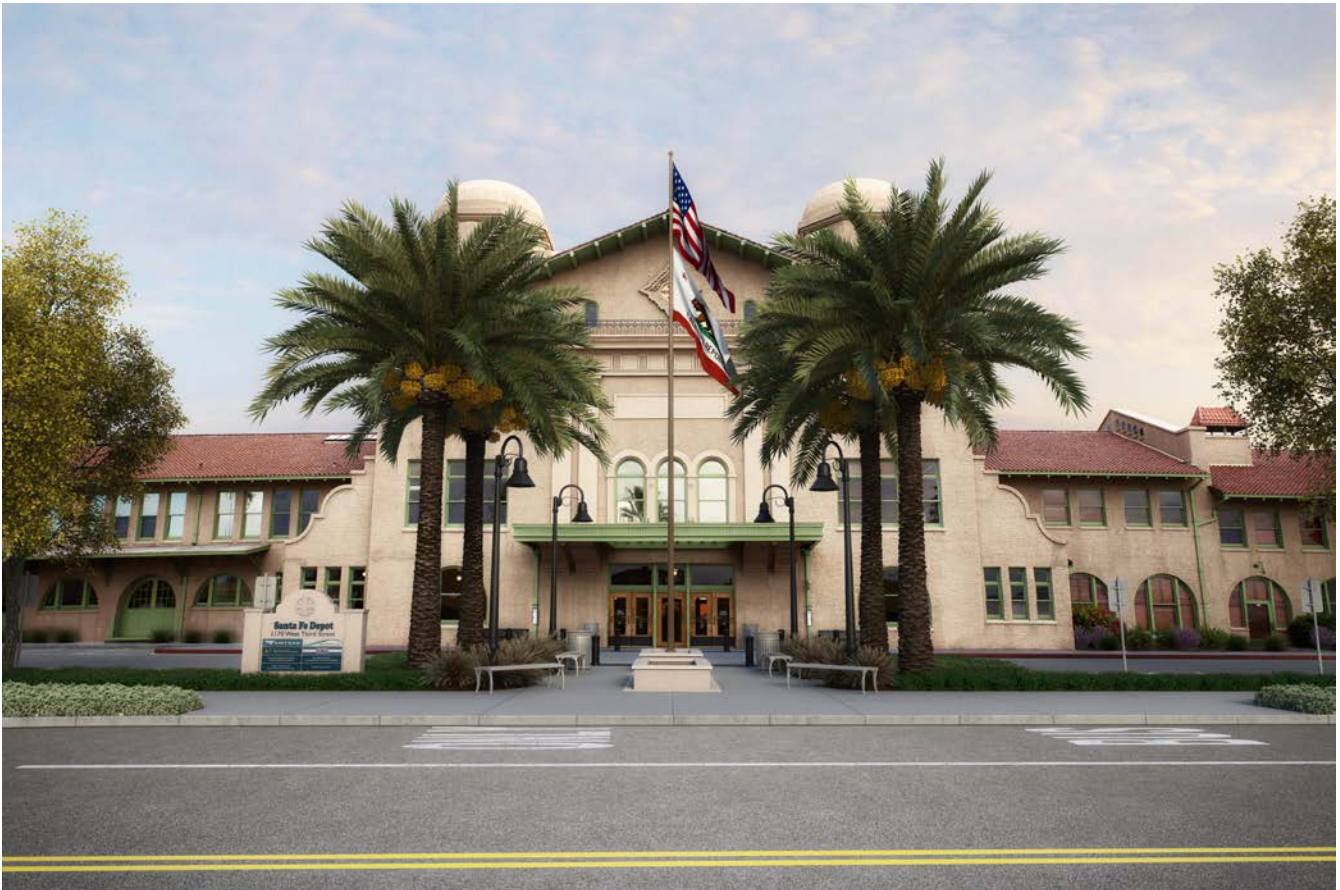
Project rendering looking at the new entrance to the Santa Fe Depot.
