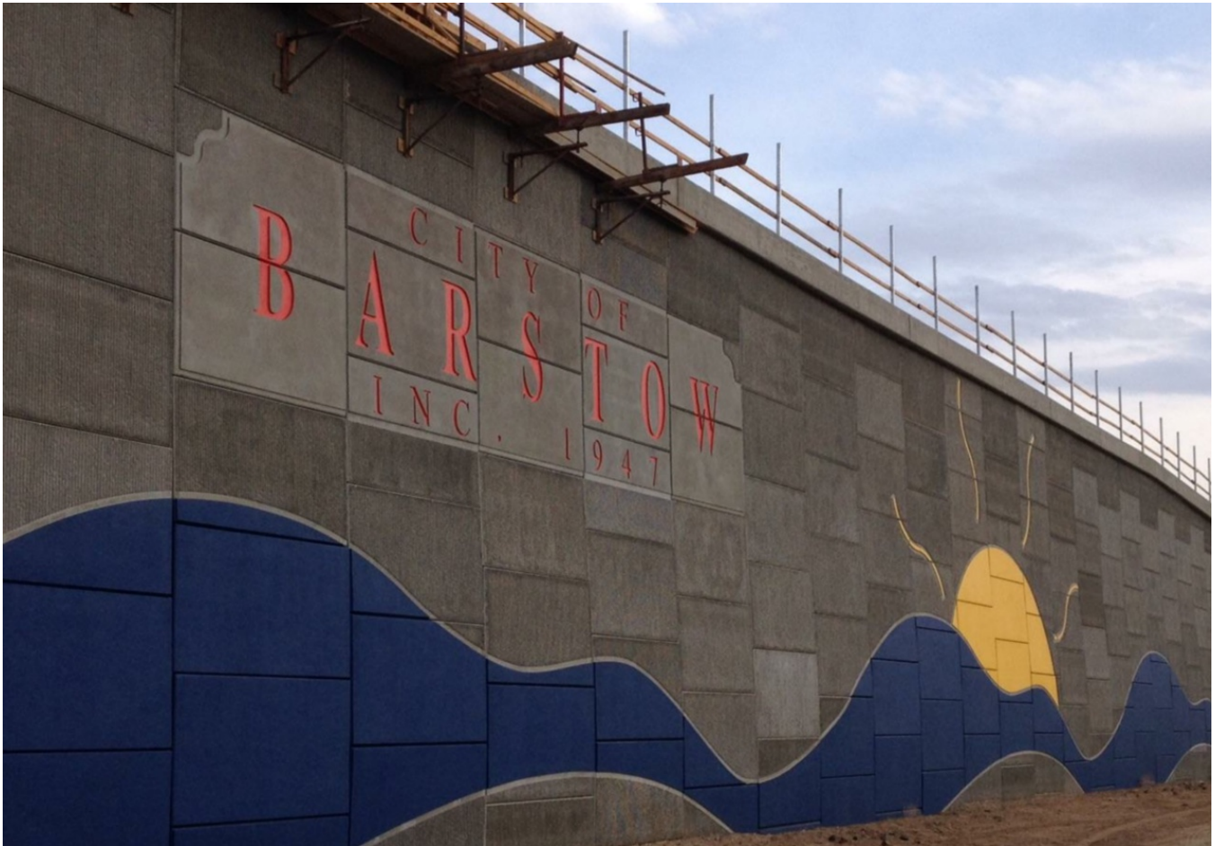
On Friday, August 21, 2015 the San Bernardino Associated Governments (SANBAG) and the City of Barstow celebrate the completion of the Lenwood Grade Separation. The project was an investment back into the region that represented our continuing rebound from the recent economic downturn.
