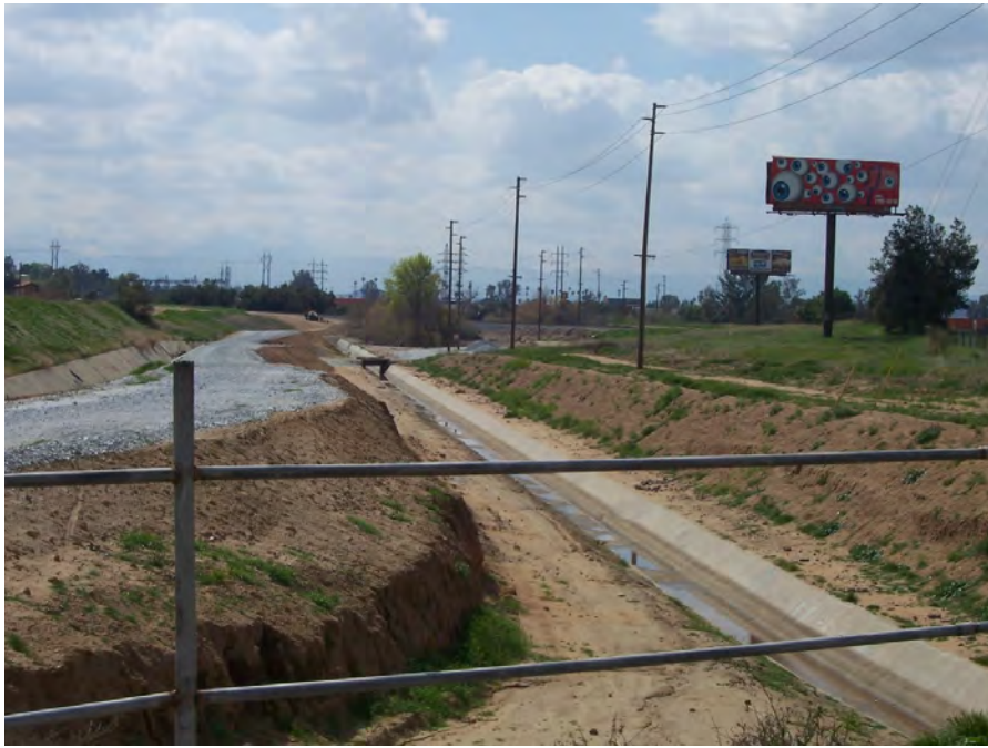
STORM WATER CHANNEL, WEST OF DEBERRY STREET, RUNNING NORTH AND SOUTH, PARALLEL TO I-215.
