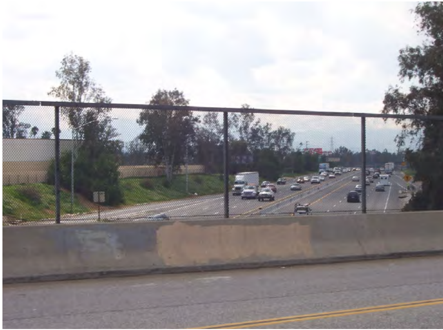
I-215 LOOKING SOUTH-BOUND FROM BARTON ROAD OVERPASS
