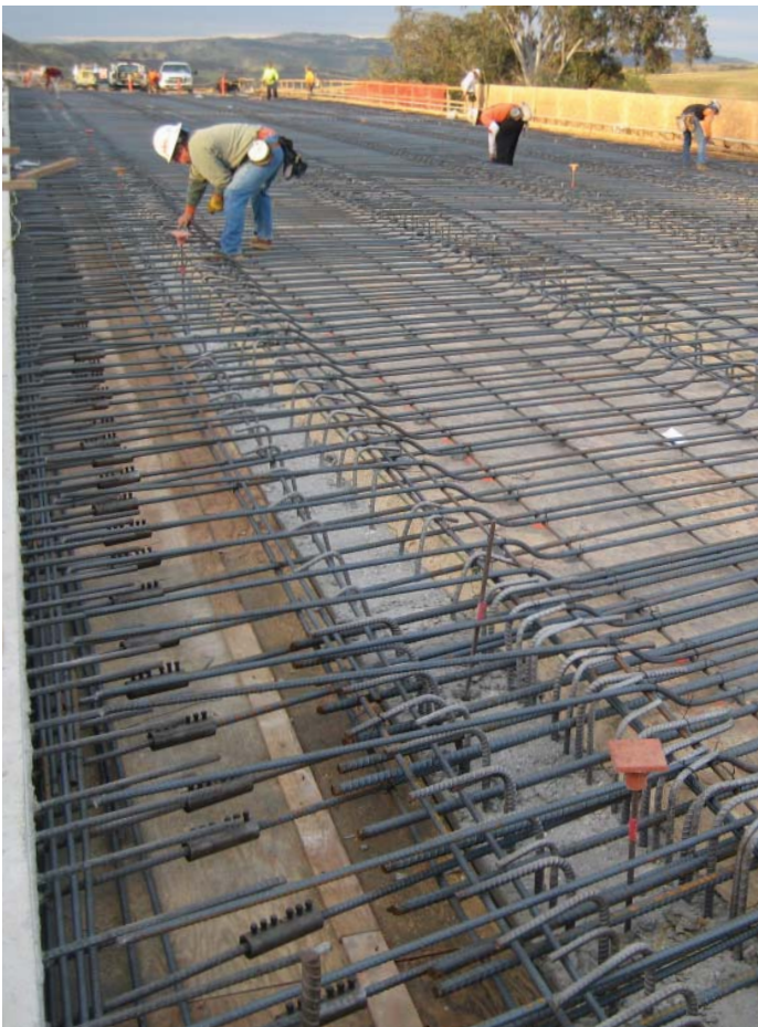
Installing deck steel
