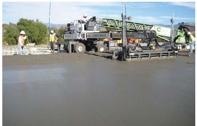
Laser screed (top) bent steel installation (bottom)
