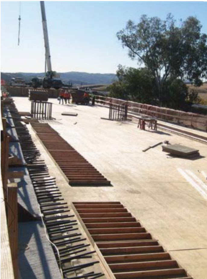
Overview of the right bridge
