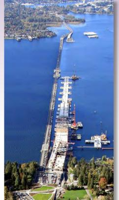
Assembling pontoons for the new SR520 floating bridge.
