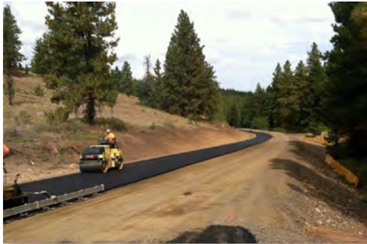
Reconstruction of McGinnis Canyon Road in Douglas County eliminated one sharp reverse curve and widened the roadway from 24 feet 30 feet. For safety, the slopes were flattened and guardrail was installed.
