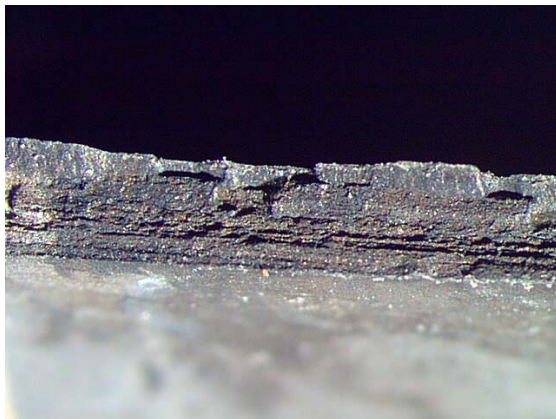
Photo 3 - edge view of Lens 21 crack
