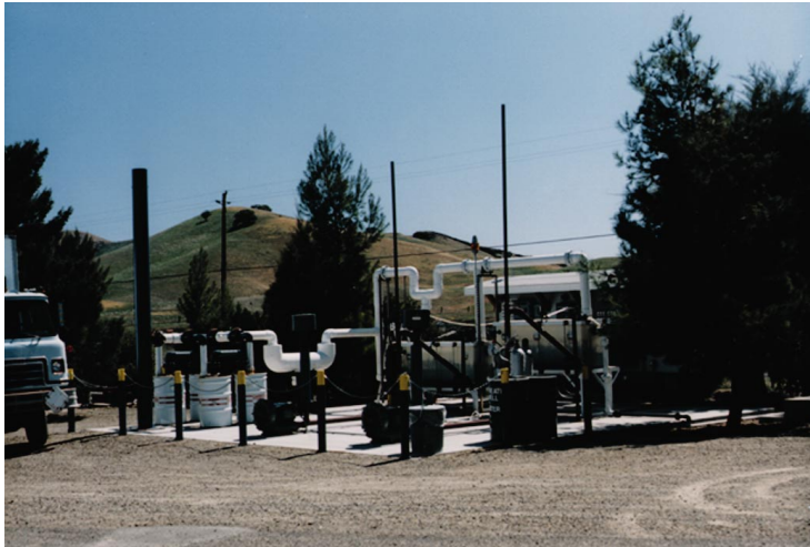
Air sparging is used to treat extracted ground water in the central GSA.
