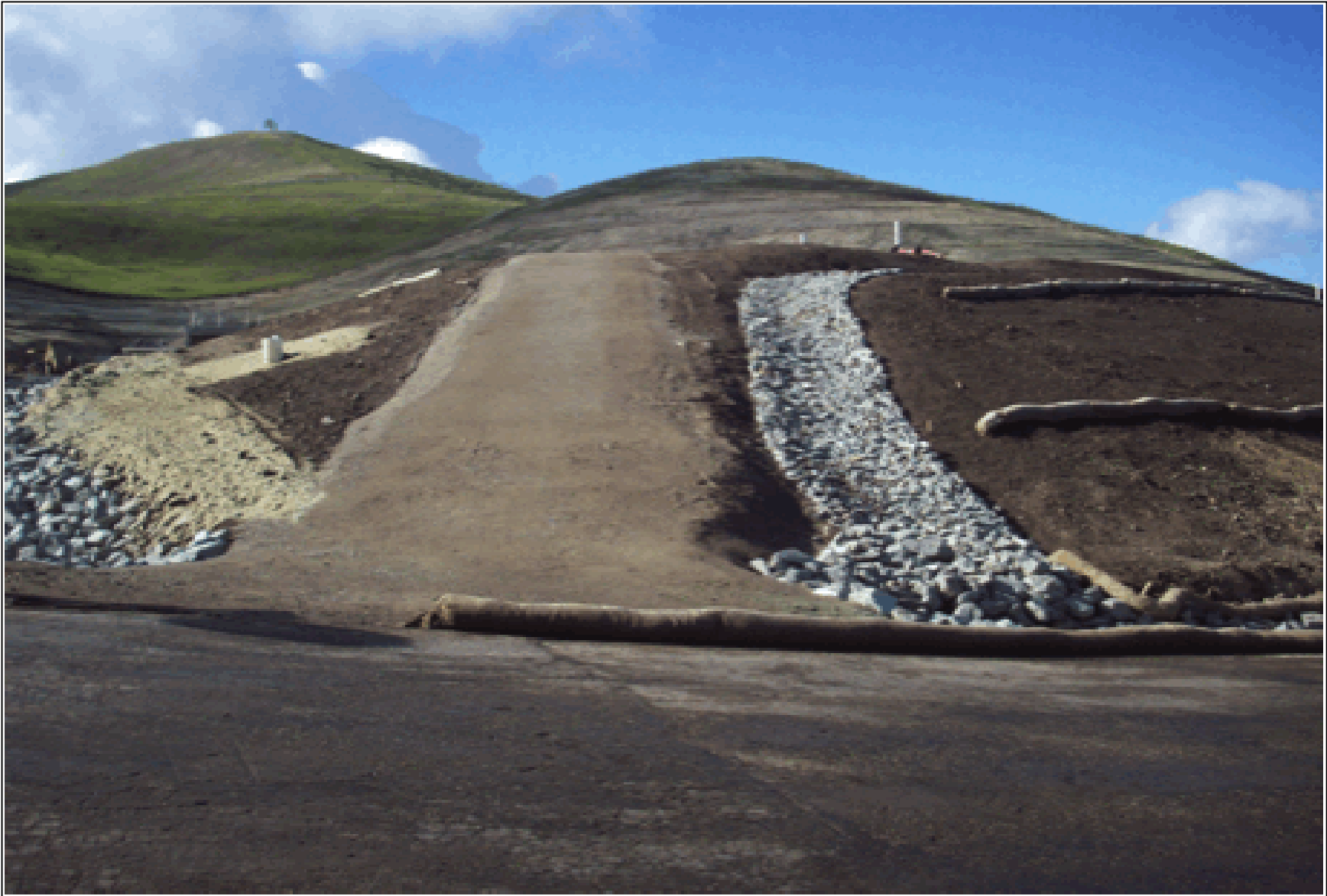
Building 850 CAMU and monitor well/maintenance access road
