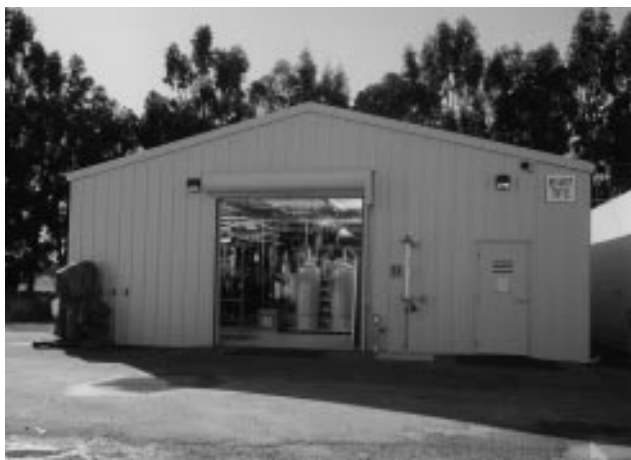
Figure 1. Treatment Facility C is designed for long term operation and is constructed inside a permanent building.
