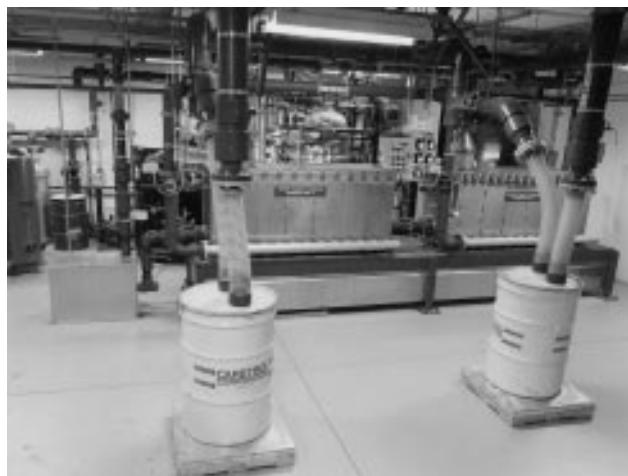
Figure 2. TFC uses air stripping to remove VOCs and ion exchange to remove hexavalent chromium from ground water.
