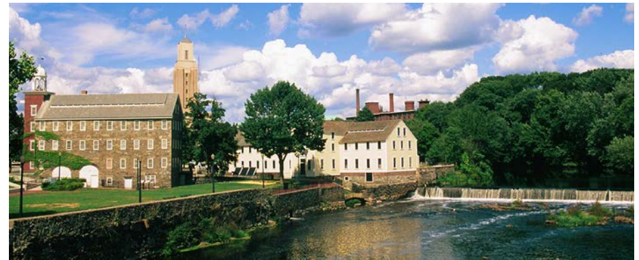
Above: Slater Mill was the first successful cotton-spinning factory in the United States. It is now a National Historic Landmark housing a museum, Jencks Education Conference Center, and Hodgson Rotary Park.
