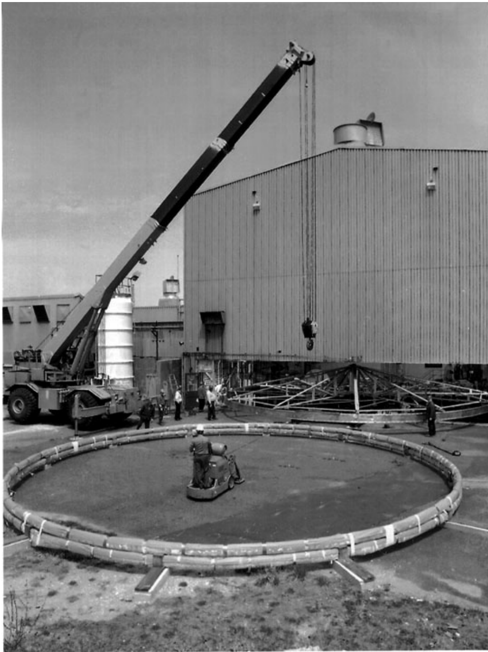
Fig. 6. The completed outer coil and cryostat were passed through the slot in the g-2 building and stored outside, in preparation for construction of the lower half of the magnet yoke. The completed inner coils in their cryostats are in the foreground.
