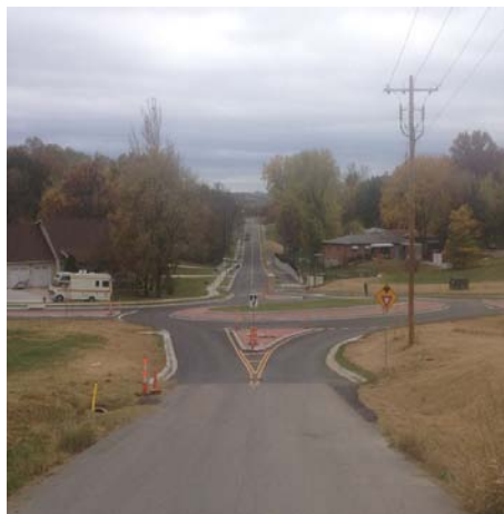
NW Road After
