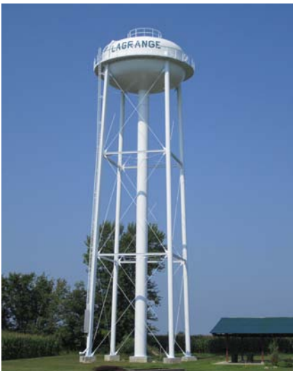
New Water Tower
