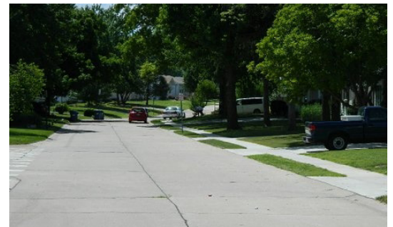
Fleetwood Sidewalk Project
